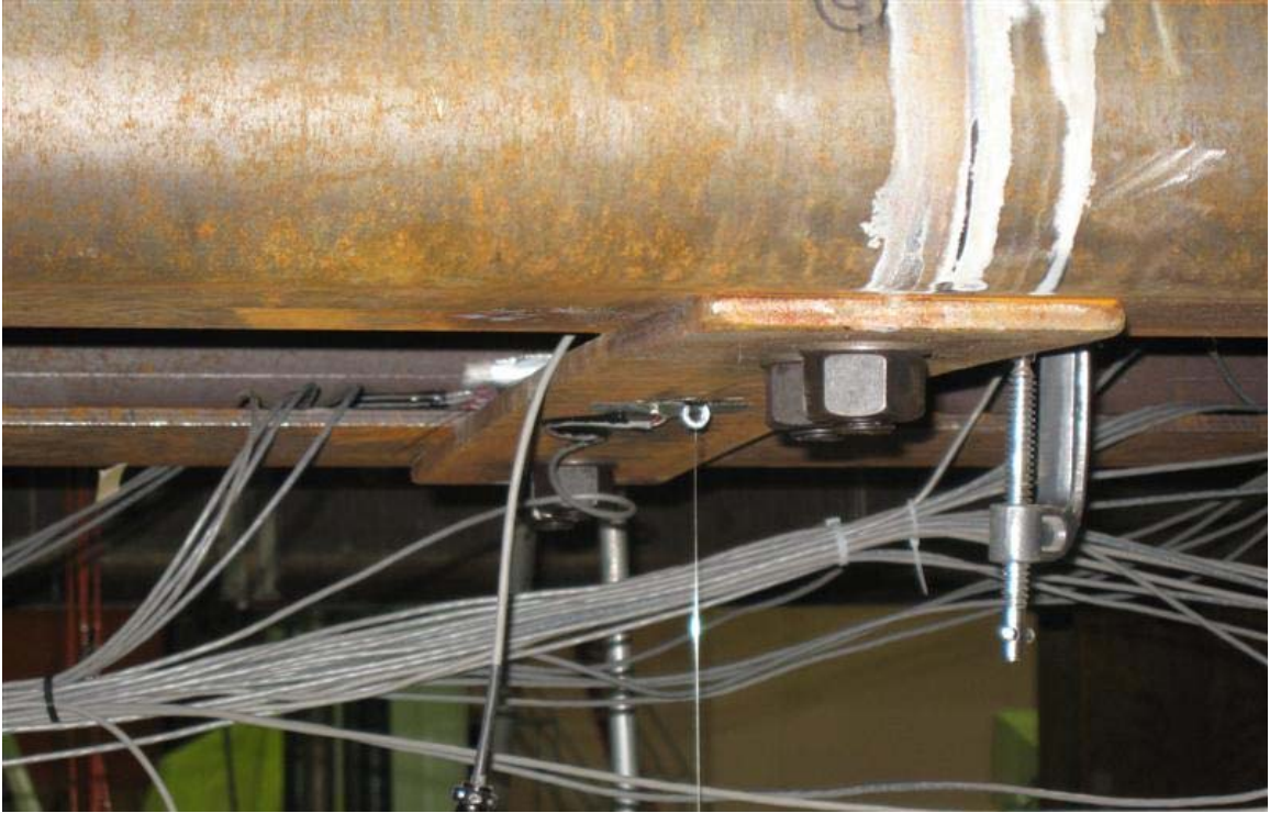
Figure 3-41 Test B1 tie plate at 140kip
