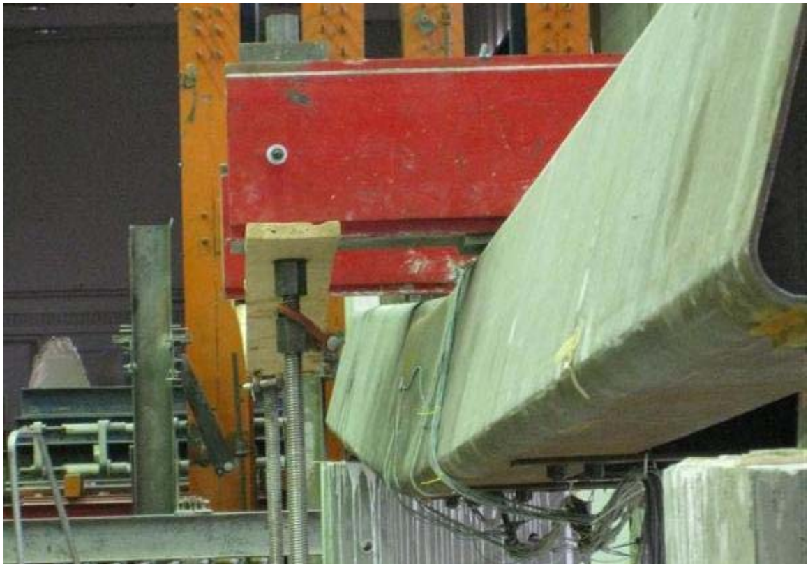
Figure 3-46 Girder deflection after unloading
