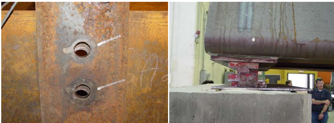
Figure 3-17 (left) Flange and tie plate bolt hole alignment after loading, (right) girder movement at support.
