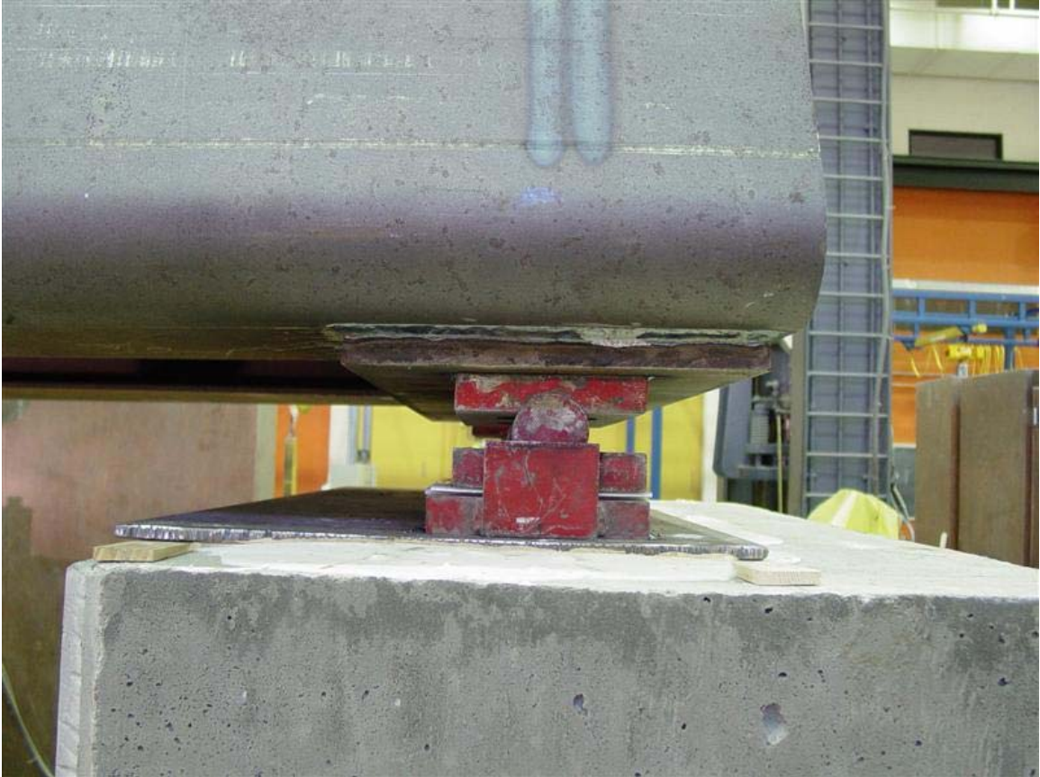
Figure 2-7 Girder bearing system
