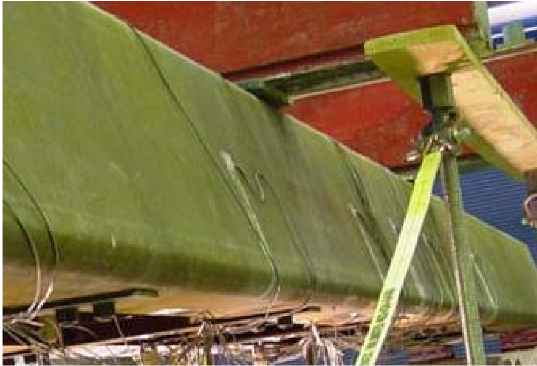
Figure 3-8 Girder web before loading
