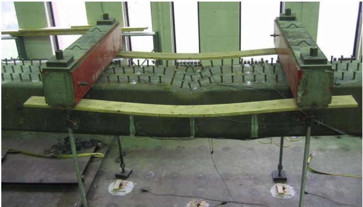
Figure 3-48 Girder deformation at midspan of girder after unloading
